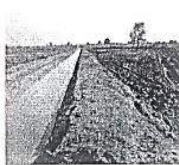
Canal position before laying HTCPM membrane
